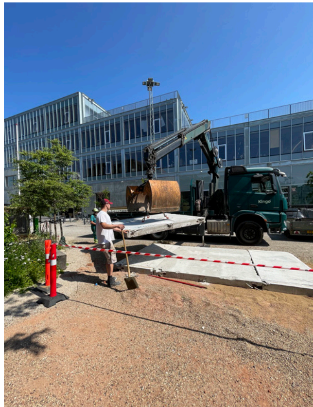
Fig 9: Konstruktion af betonplatformen. / Assemblage of the concrete platform foundation.
