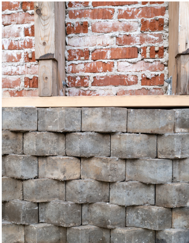
Fig. 14: Møde mellem forskellige materialer og konstruktive systemer / Connection (transition) between different materials and construction systems
